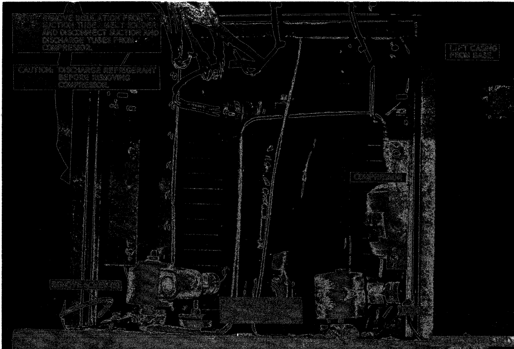
Figure 5-10①. Compressor/motor assembly, removal and installation.
